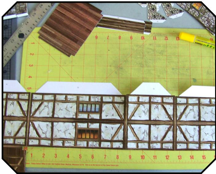
3: Glue the four wall sections as shown above (alternate wall lengths; 4"-8"-4"-8"). Do this for both floors.
