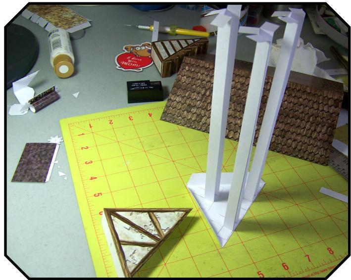
2: Glue the three support beams to the inside of a roof end as shown above.
