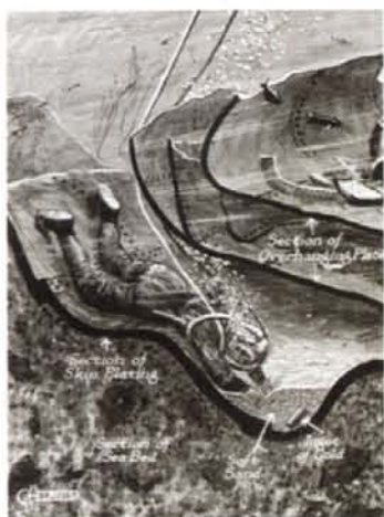
ABOVE: The top illustration shows diver Light blown up feet first while working on the wreck of the Laurentic . This was likely to happen if the air pumped down to the diver was at a greater pressure than the surrounding water. The illustration below shows one of Captain Damant's divers digging down for gold.
