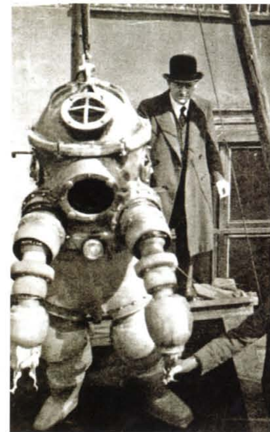
ABOVE: This 'iron man' diving suit proved too cumbersome for practical use, something that became apparent to Captain C. Wilson (right), who led two or three expeditions in search of the Tubantia 's gold in the 1930s.
