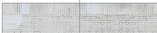
Internal plinth cover layers
