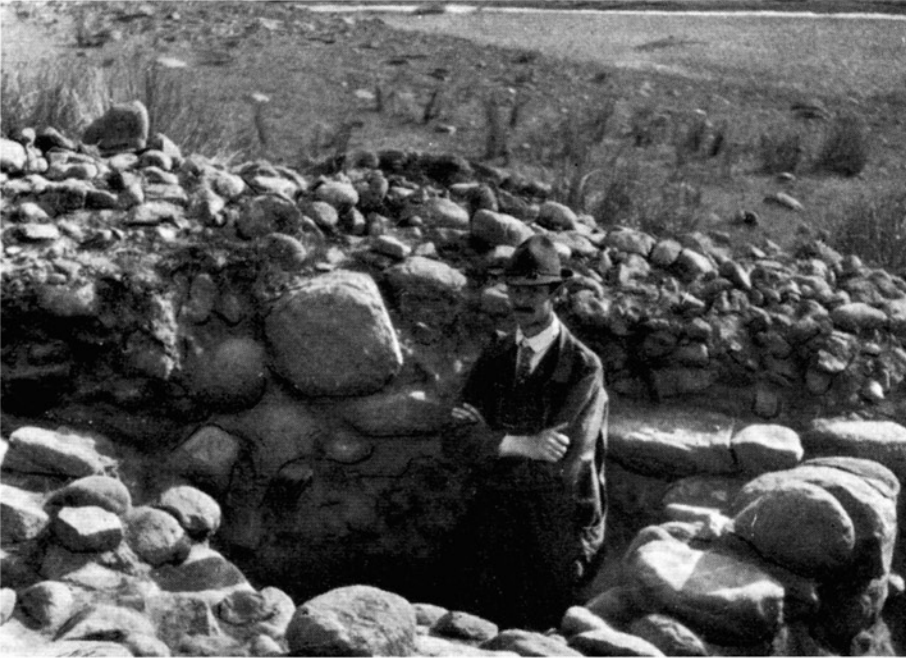
A worker stands in one of the post holes which Schulten discovered on the Numantia siege wall south of Dehesilla. The hole is elliptical, 4½ft (1.3m) long by 2½ft (0.8m) wide and 5¼ft (1.6m) deep. Schulten reasoned that the large dimensions were to allow a thick upright timber to be securely wedged in place. (A. Schulten, Numantia: Die Ergebnisse der Ausgrabungen 1905–1912 , vol. III: Die Lager des Scipio , Munich 1927)
