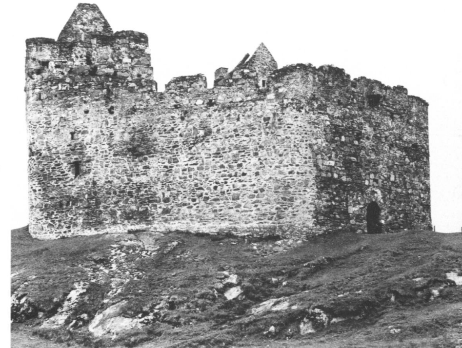
16 Castle Tioram, Loch Moidart, Argyllshire. The lofty, thick curtain wall was largely defended from the battlements, either from the little box machicolation sticking out over the entrance gate (on the right) or from projecting timber hoards (now gone) supported on timbers placed in the putlog holes (visible near the wall-top).
