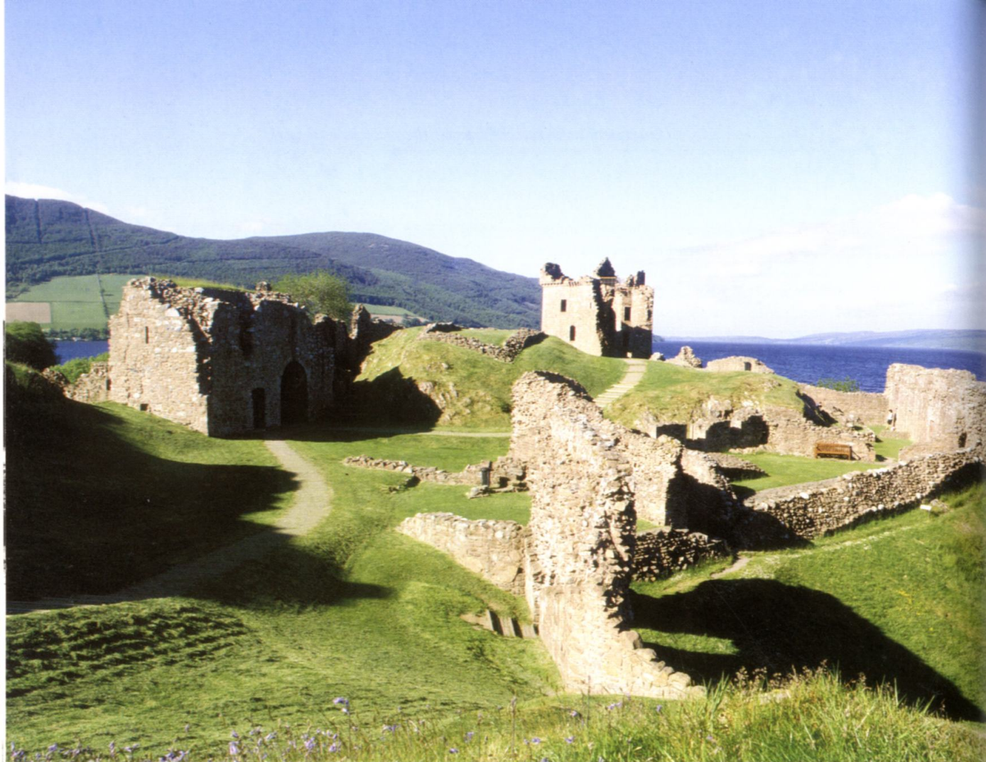
72 The sixteenth-century Grant Tower dominates the sprawling castle at Urquhart, beside loch Ness.
