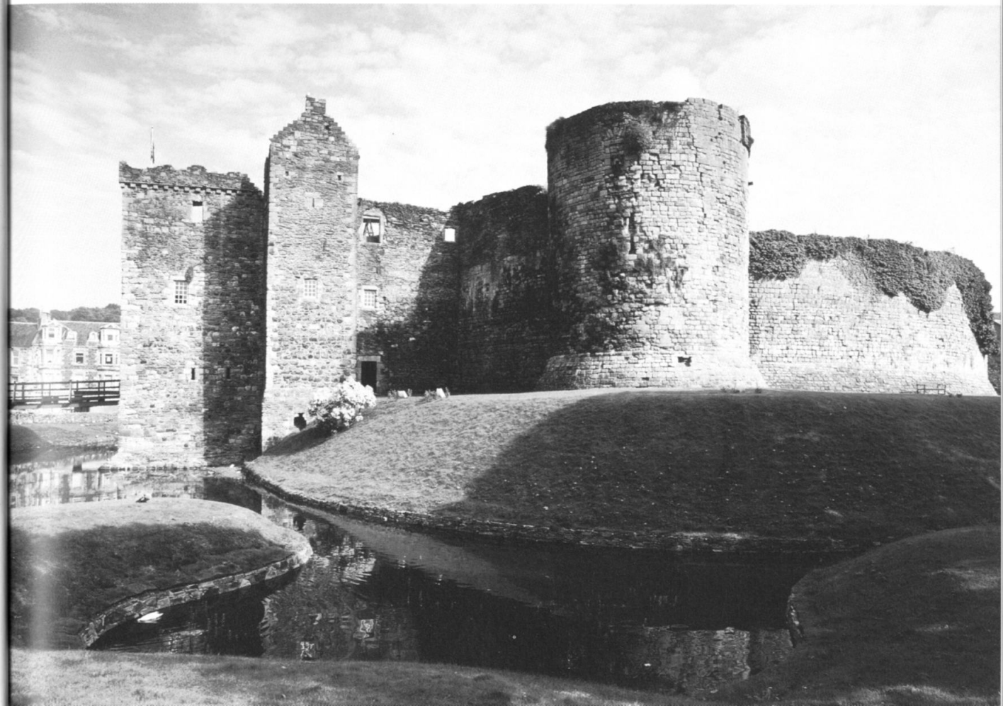
19 Rothesay Castle, the Stewart stronghold on Bute. The original circular curtain wall, built about 1200, was furnished with projecting round towers, a battered wall base and crenellations in the later thirteenth century. King James IV added the imposing gatehouse on the left about 1500.
