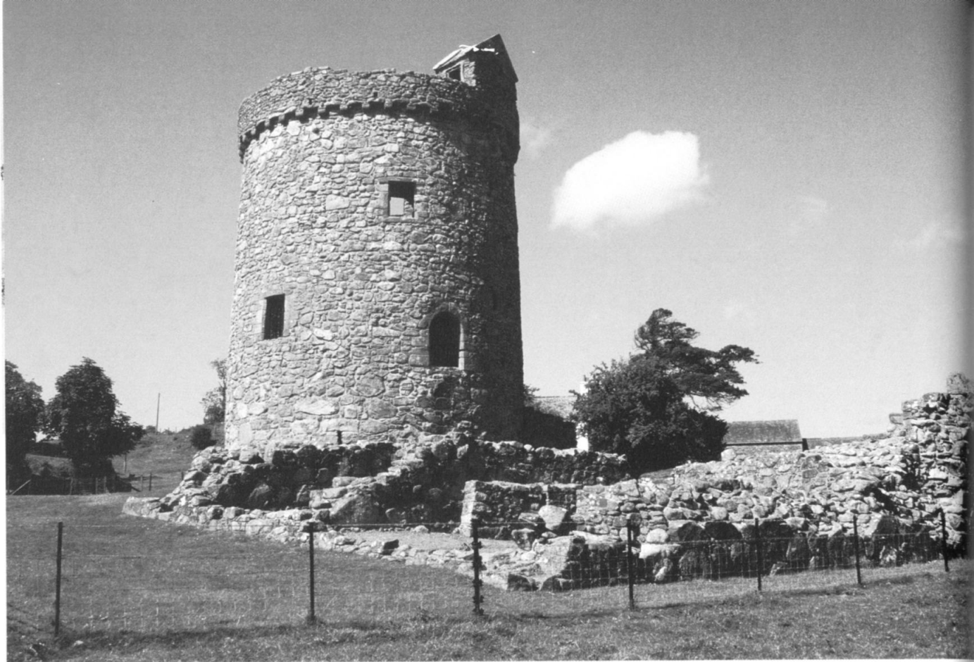
51 Orchardton Tower, the residence of the Cairns family near Dalbeattie, Kirkcudbrightshire. The tower's circular shape is unique in Scotland, but in most other respects the castle complex is typical. The round-headed doorway a third the way up the tower gave access between the laird's apartment and the more public outer hall in the foreground.
