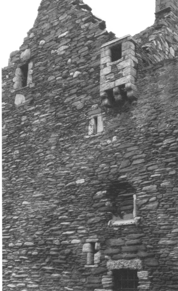
59 The box-machicolation projecting from the front wall of Lochranza Castle, Arran. This simple device enabled the defenders to protect the entrance door below.
