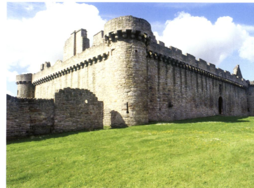
58 The inner curtain wall at Craigmillar Castle, Edinburgh, with its attractive machicolated parapet and projecting round towers fitted with gunholes.
