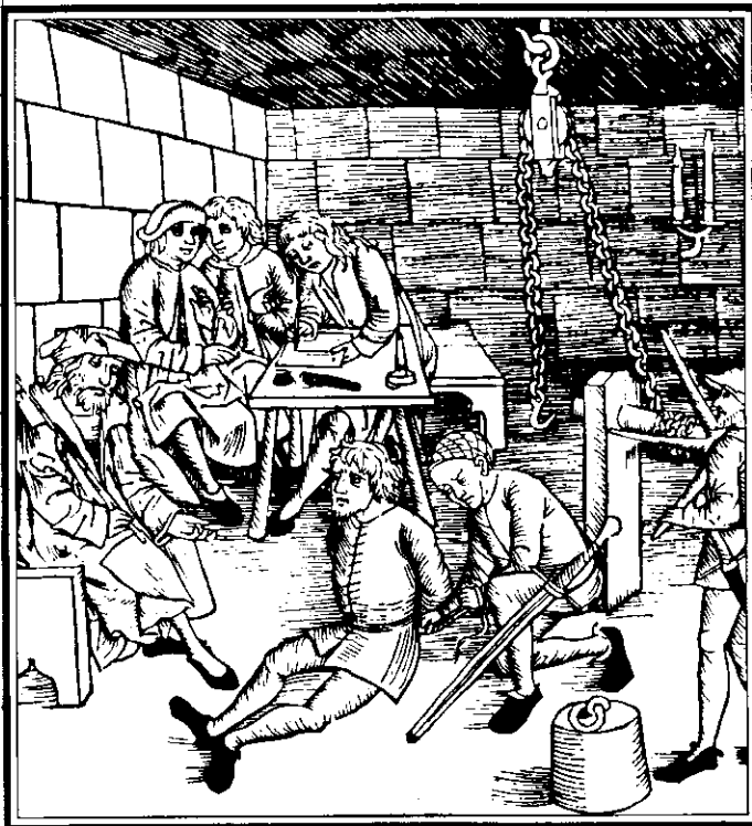
Wrong-doer being prepared for 'painful interrogation'.
